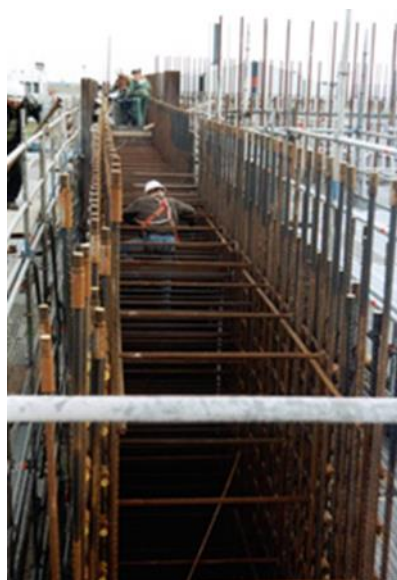
Figure A.5 Worker at work in a concrete 1.7 m thick outer wall
