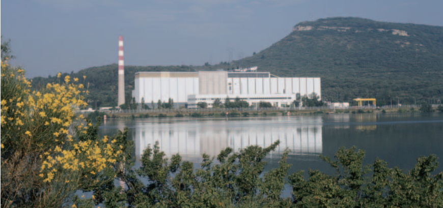
Fig. 14: Phénix sodium-cooled fast-neutron reactor in Marcoule (France)
