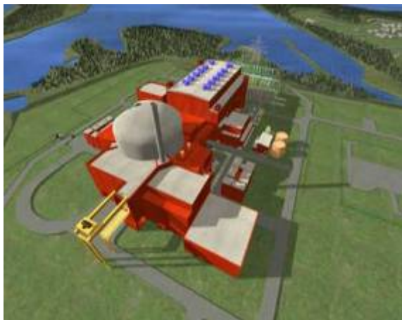
European Pressurized Water Reactor
