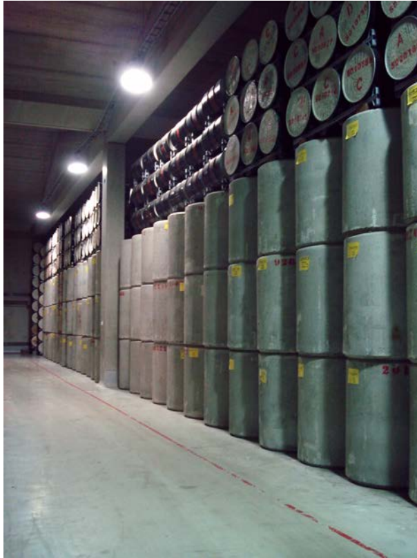
FIG. 2. Storage facility for LILW.
