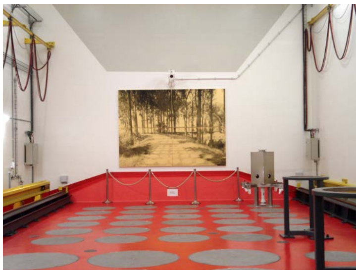
FIG. 3. Storage facility for HLW.
