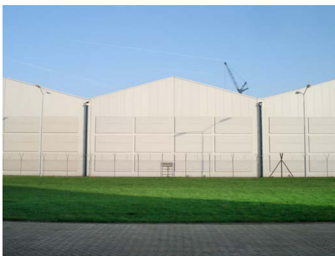
FIG. 4. Storage facility for NORM waste.
