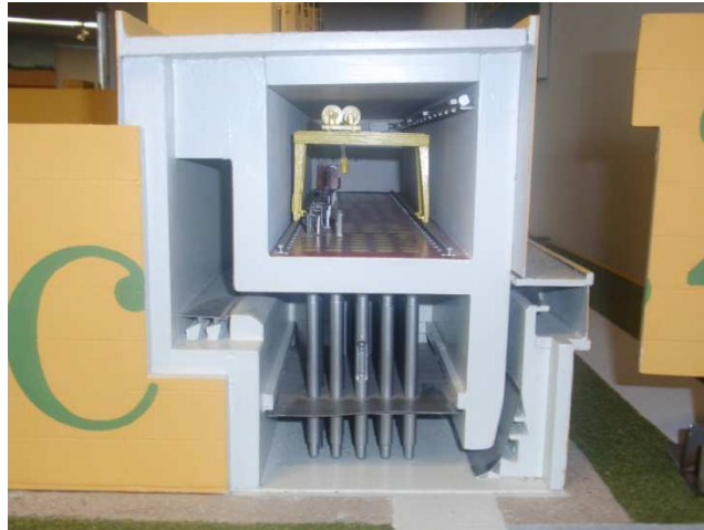
Figure 1.14 Cylindrical wells for storage of HPW (scale model)
