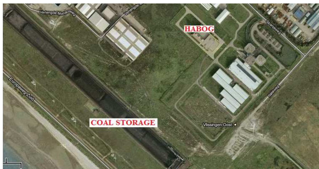
Figure 6.4 Location of the coal storage
