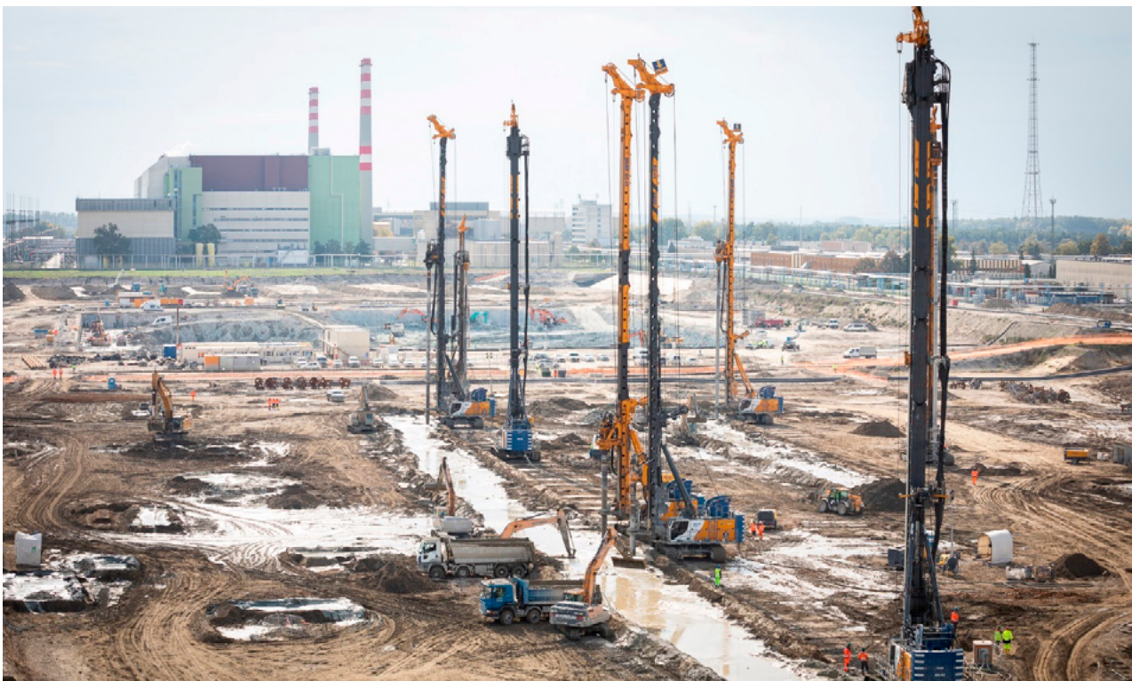
The Paks II NPP construction site in October 2024. The units of the operating Paks NPP are visible in the background, and in front of them is the excavation pit for the first unit of the Paks II NPP (or the fifth unit of the entire Paks NPP). Photo source: Facebook Paks II. Atomerőmű Zrt 157 .
