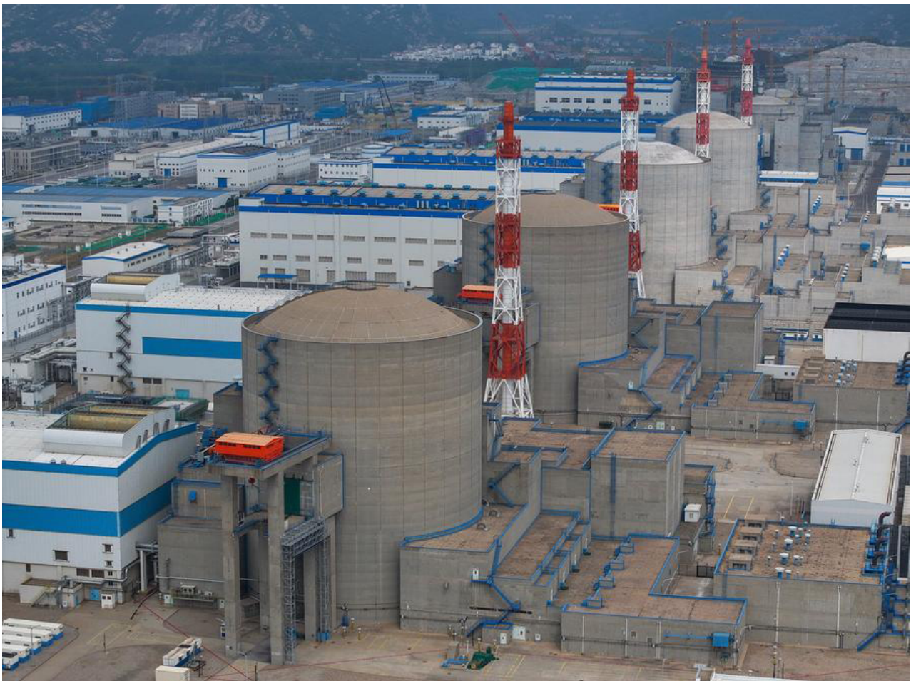
Tianwan Nuclear Power Plant, 2024. In the foreground are the first four Russian-designed VVER-1000 reactor units. Source: Xinhua/Li Bo
