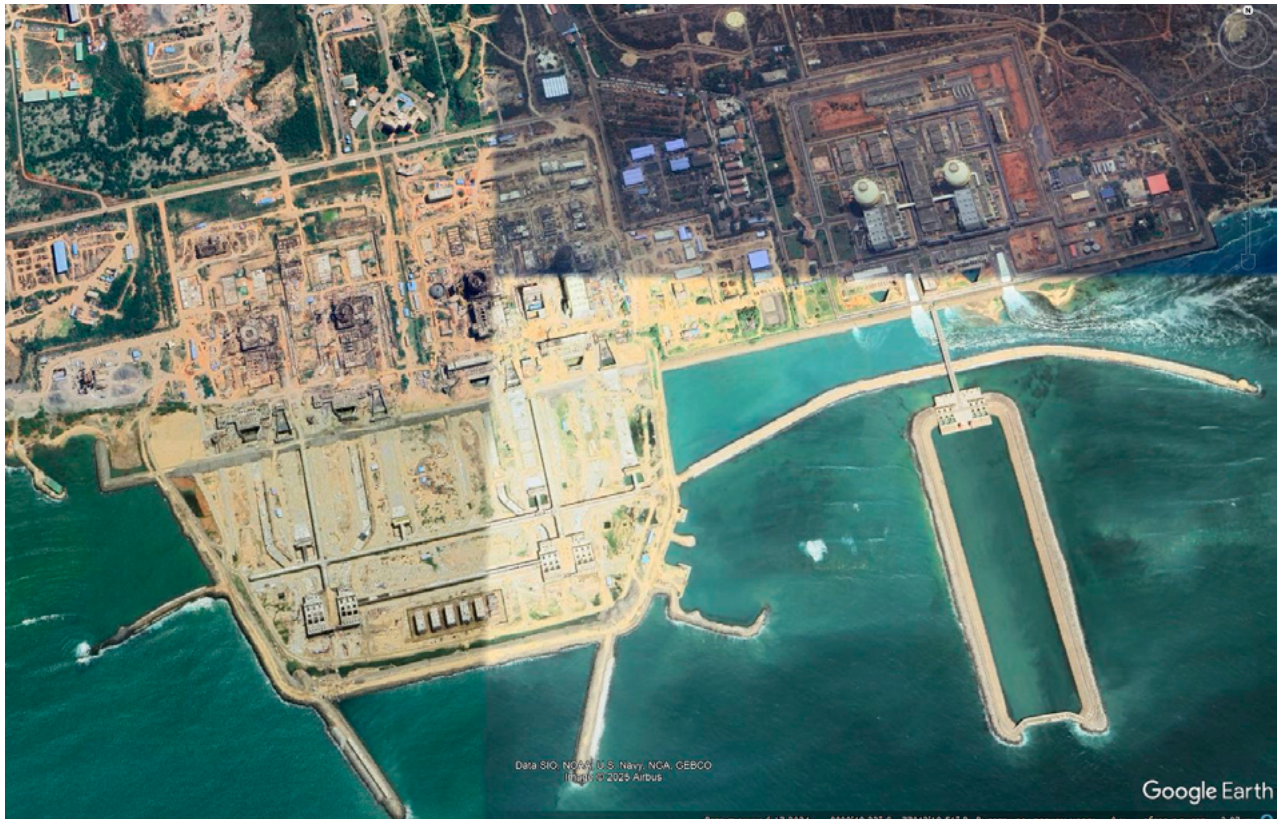
Satellite image of the Kudankulam NPP site in summer 2024. On the top right are the two operating units № 1 and № 2. On the left are units № 3-№ 6 under construction. Source: Google Maps.
