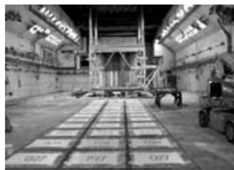
indicated by the covered circular openings. Right: Inside the U.S. K-Area Material Storage Facility at Savannah River, constructed in the reactor hall of a decommissioned production reactor. Pallets with plutonium containers are to be stacked inside the room shown.
