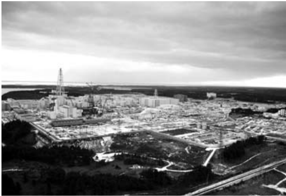
Figure 1.10. The Rokkasho Reprocessing Plant. [Source: Greenpeace/Gavin Newman]
